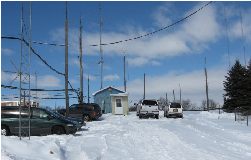
The Shack in the Farm (more antenna's then a porcupine)
